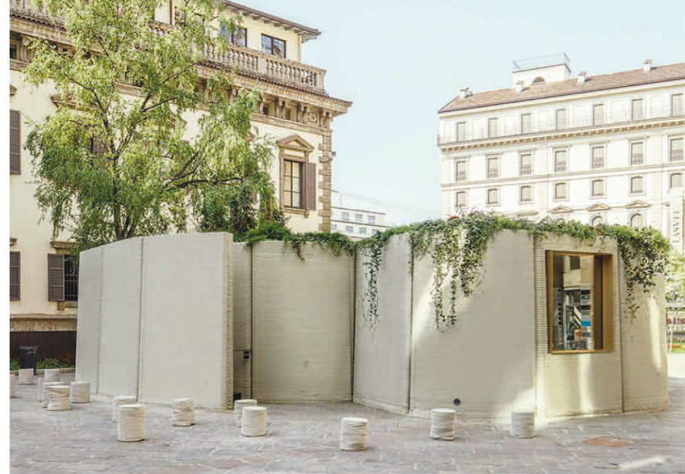
The roof garden is reached by means of external stairs. Usefully, some climbing plants can adhere to the corrugated wall without any other support. The title of the project – 3D House 05 – refers to the five key criteria on which the build is based: creativity, sustainability, flexibility, affordability and rapidity
